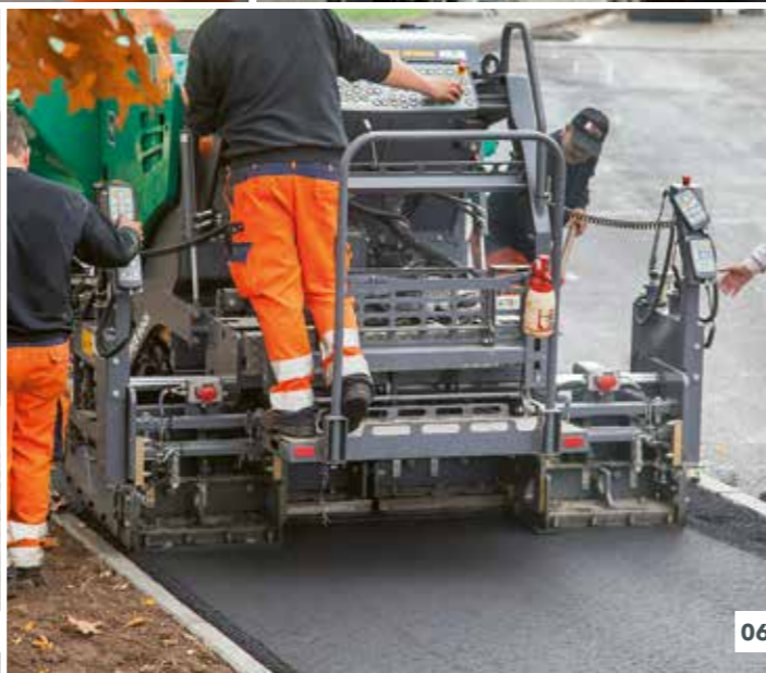
04 All the key paving functions can be controlled by the two handy remote control units for the screed. 05 Niveltronic Basic fully integrated automated grade and slope control. 06 Can be combined with the AB 200 and AB 220 Extending Screens.
